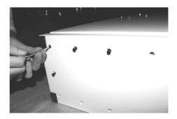
11. Pull the three pairs of cables through the holes in each cabinet bracing.
